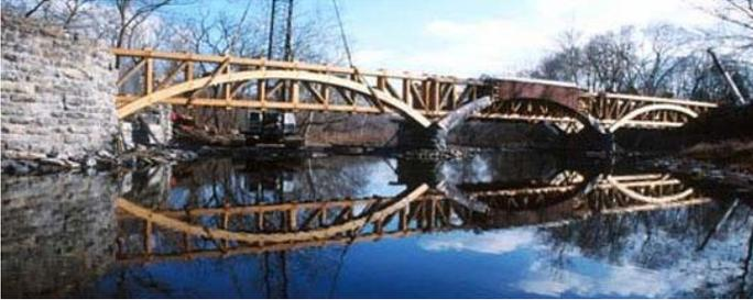
The patent addresses a common problem of conventional glued-laminated beams, which is that they often fail in bending-induced tension. The Advanced Structures and Composites Center has found that adding small amounts of reinforcement to the tension side of the beam significantly increases its strength.
